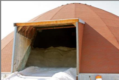
Salt storage dome in Philadelphia, PA
