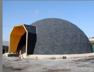
Salt storage dome in Baltimore, MD
